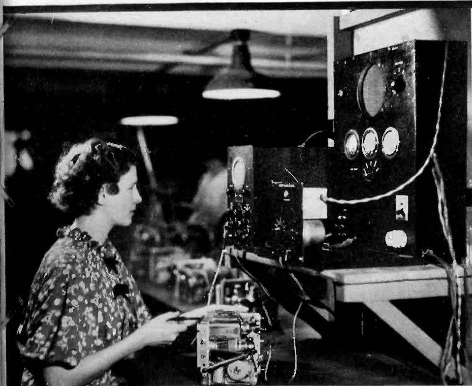
6 Automobile receivers—another huge annual market—are aligned here by a cathode ray tube
