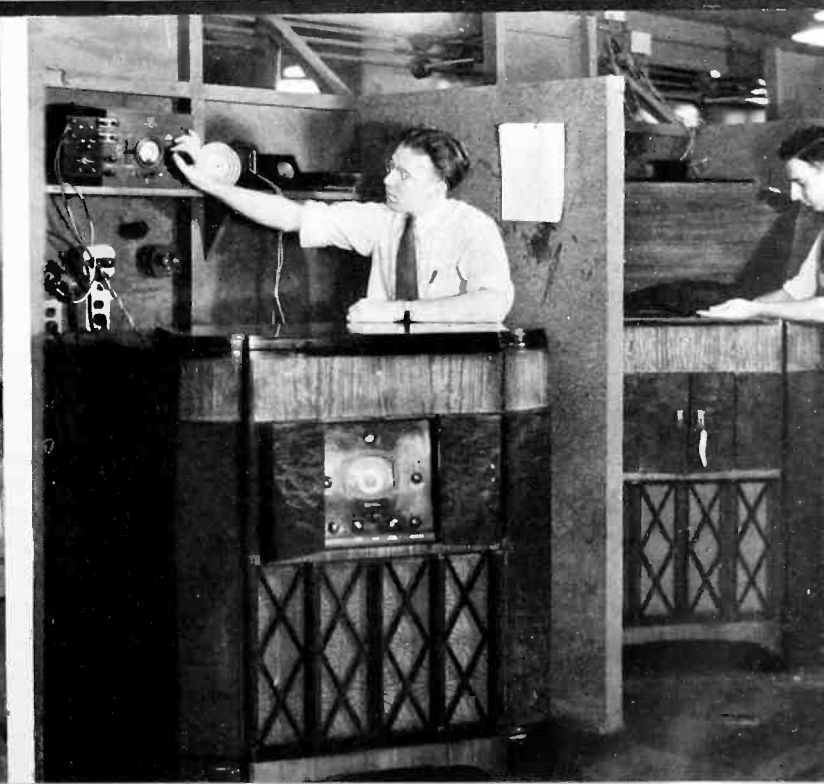
7 A final assembly test. Even after this, a few sets are picked at random at the shipping room
